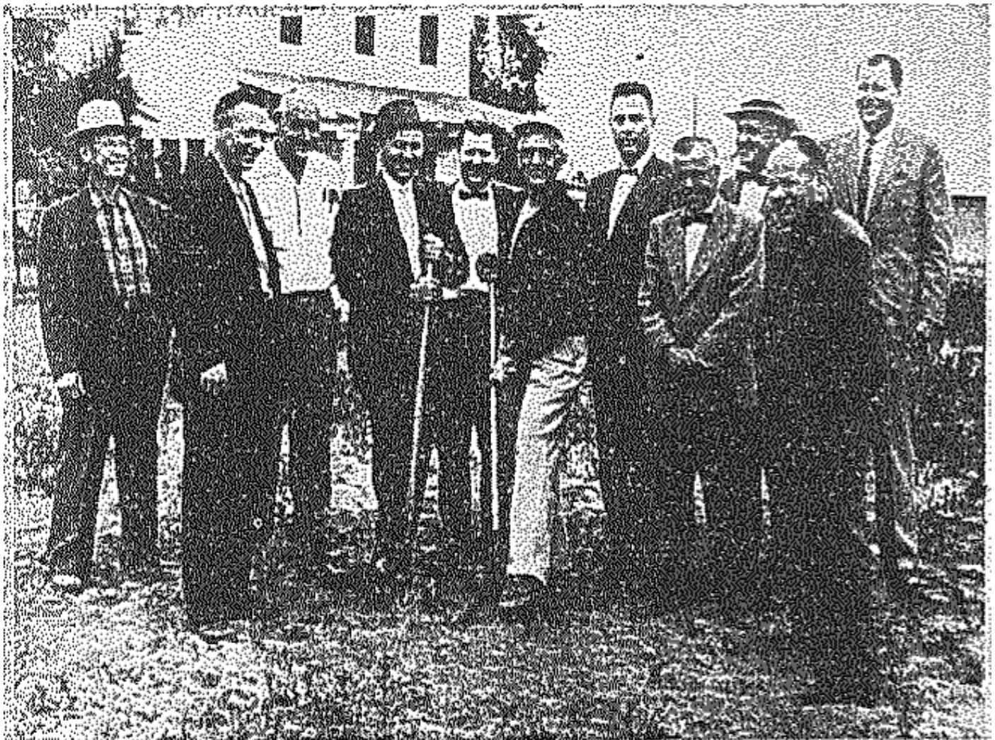
AT GROUND BREAKING — Ground was broken Thursday in Chula Vista for the first Food Midget Market — one of 20 planned — with officials of the company taking part at the Broadway and K street site. Pictured here are Ed. Culnan, Rex Mounts, Ed Loustalot, Nathan
