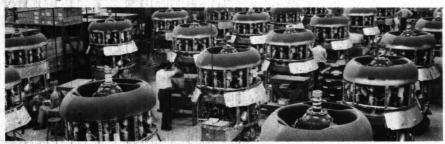
Power Packs for B-24 Liberators during World War II, 31,700 units were manufactured by Rohr Aircraft.
