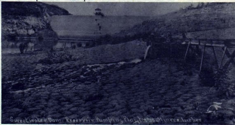
Sweetwater Dam. Reservoir Pumping Plant. (San Diego County Archives)
