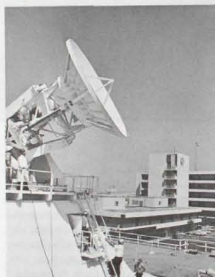
High precision millimeter wave radio-telescope built by Rohr for Aerospace Corporation and seen in operation atop one of the Aerospace buildings at El Segundo, Calif.
