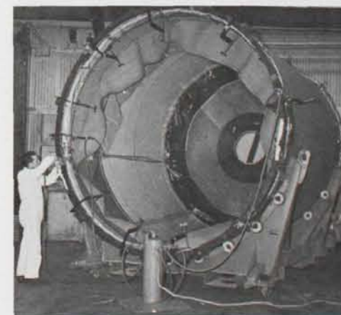
Locating tools for use in bagging an insulation segment for United Technology Center's 120-inch rocket motor case. The case is completely insulated in the propellant area.
