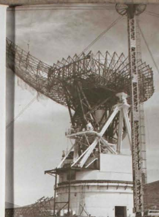
Construction proceeds steadily with the installation of radial rib back-up structure on the giant 210-foot tracking antenna, largest of its type in the free world, designed and being built by Rohr Corporation for the Jet Propulsion Laboratory.
