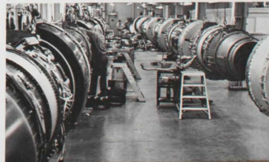
Power plant build-up for Boeing jet transports on the long monorail lines at Rohr's Auburn, Washington plant, only a few miles from Boeing Commercial Aircraft Division facility at Renton, Washington.
