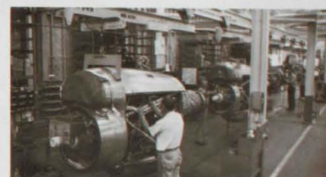
P-3A Orion propjet power packs on the monorail engine line at Rohr-Chula Vista.
