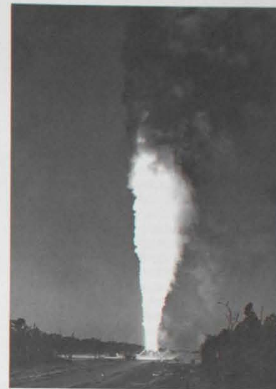
The nation's largest and most powerful space booster demonstration motor, developed and test fired by Thiokol, generated three million pounds of thrust.
