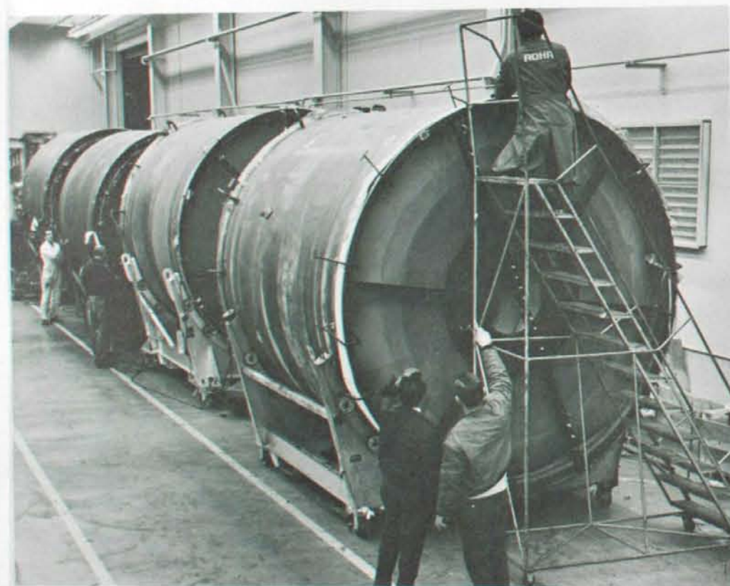
Motor cases for the United Technology Center's 120-inch solid fuel Titan III-C strap-on boosters being insulated at the Rohr Space Products Division.
